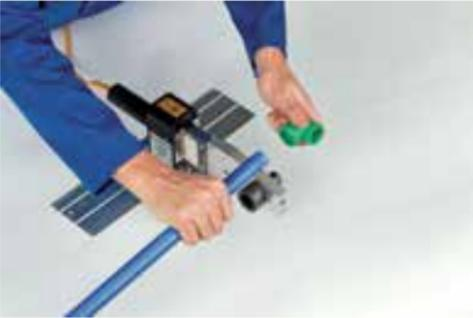
Load both the pipe and fitting on to the adapter simultaneously. Stop inserting the pipe when the mark reaches the edge of the socket and the fitting stops at the raised shoulder of the spigot.
