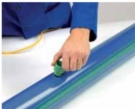
There is no DVS heating time for a fusion outlet. Once fully inserted, look for a 360° visual indication of melt (bead) on both the fitting and the pipe.
